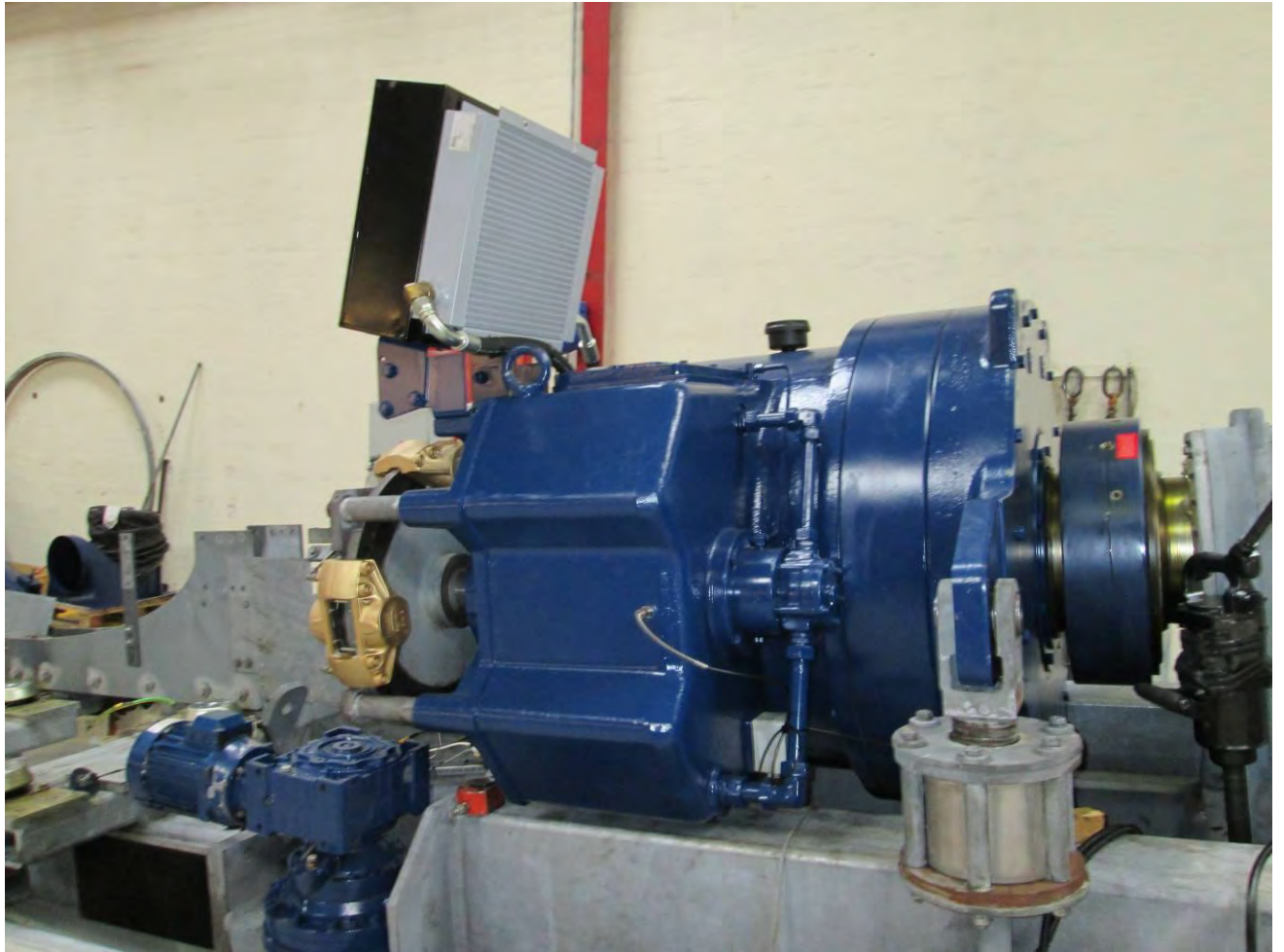
Gearbox mounted in the turbine.
