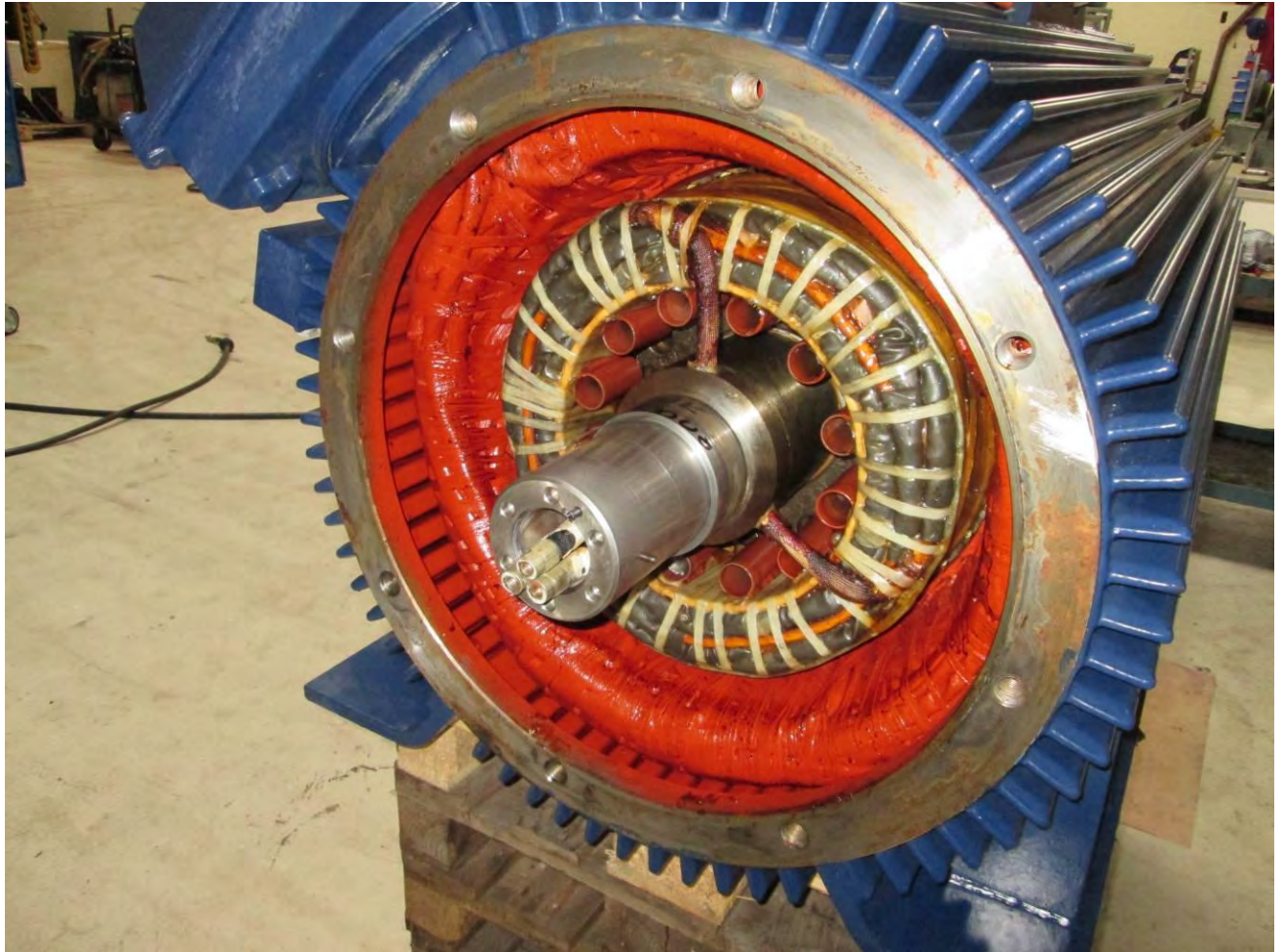
Bearing exchange generator NDE
